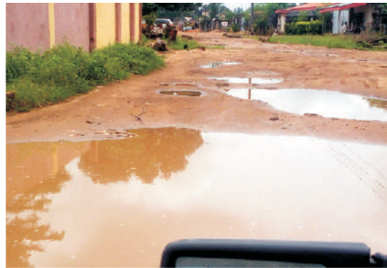
Plate 4: A flooded street with blocked gutters
