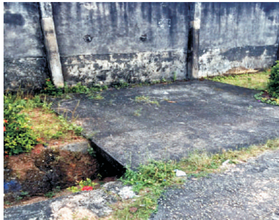
Plate 27: Water supply outlets from a residence
