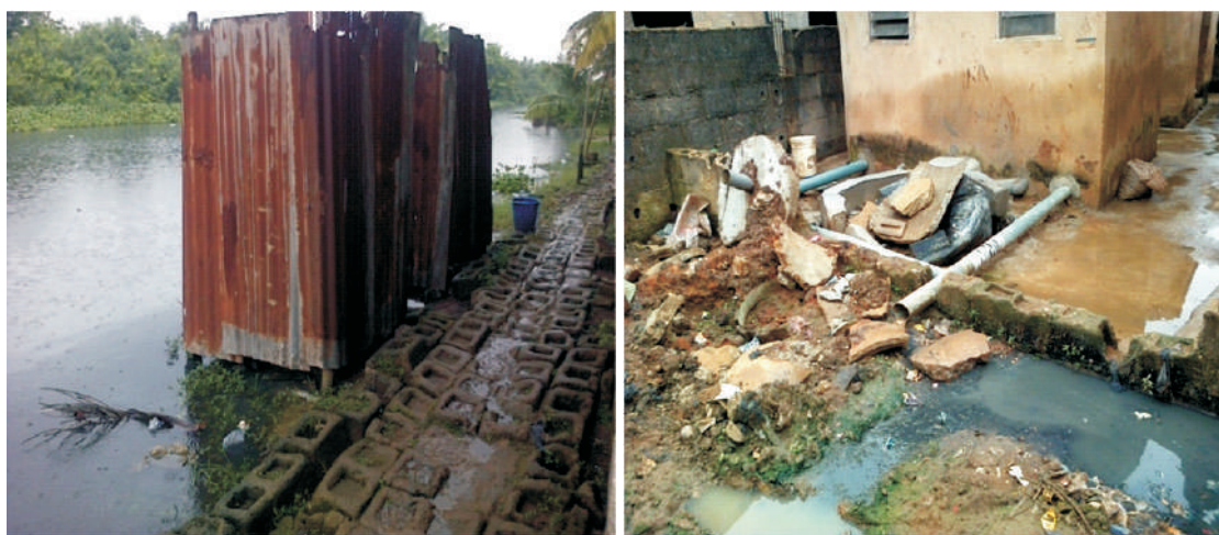
Figure 3: Toilet and bathroom built on a river
